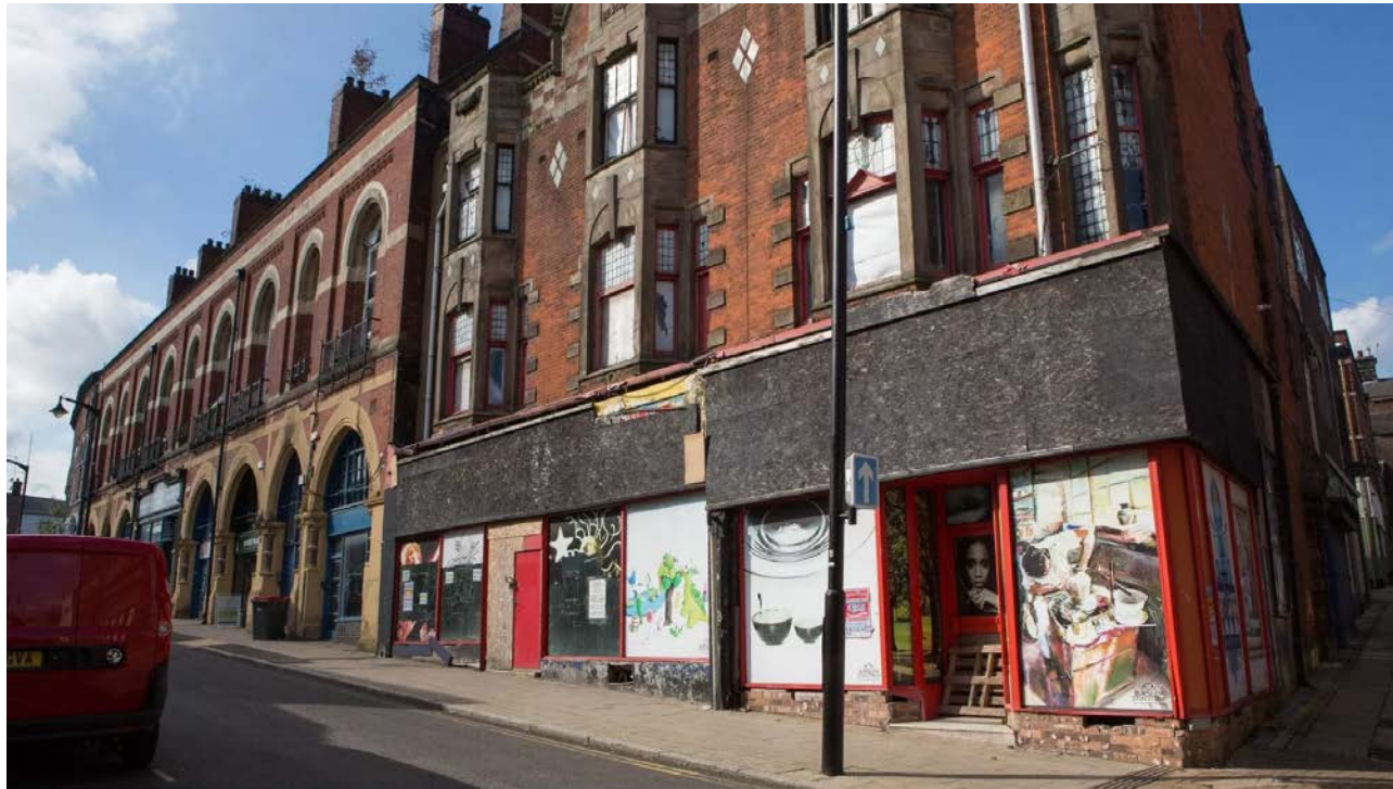
Derelict high street, Stoke-on-Trent, UK
